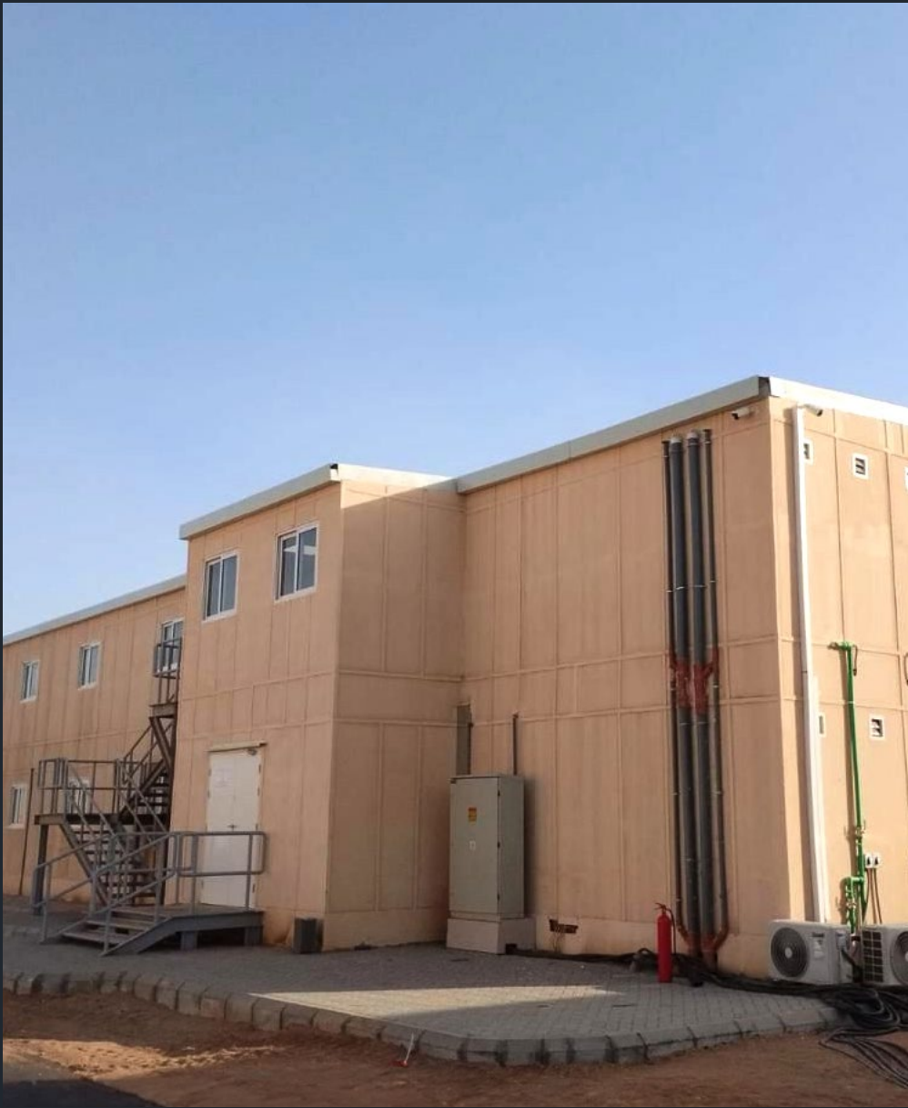
THE RED SEA PROJECT KSA - OFFICE BUILDINGS
