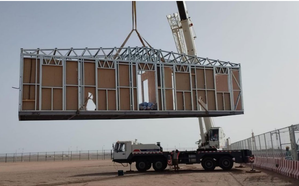
THE RED SEA PROJECT KSA - OFFICE BUILDINGS
